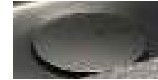
BRANDED OVERLYING STAINLESS STEEL DRAIN COVER
